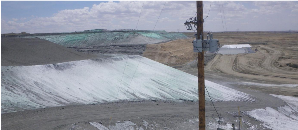
Figure 19: Fly Ash Pile (back) next to single-lined pond (left) with dust-suppression (white) and pH adjustment (green).
