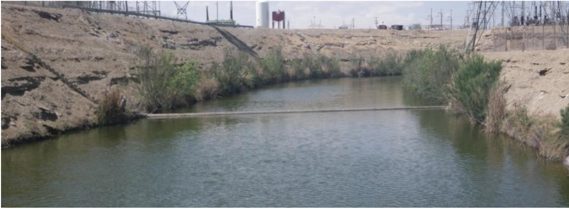
Figure 8: Berm wall before intake channel to draw only bottom water from Lake Morgan.
